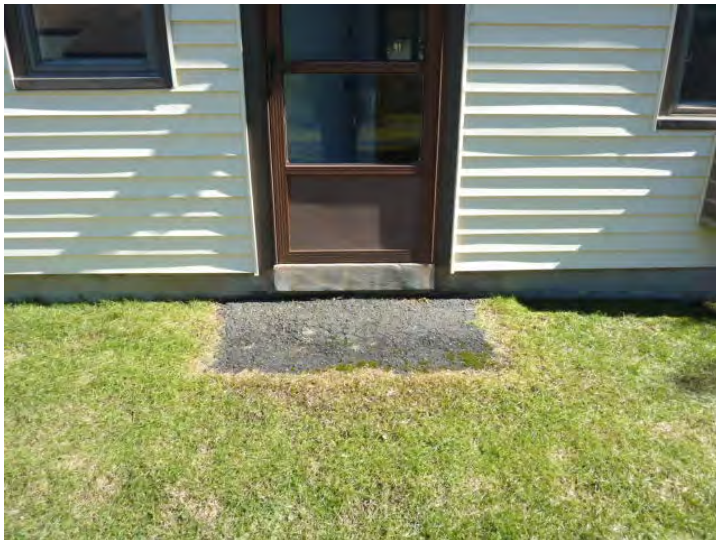
Unit and screen doors have failed finishes and are well worn. At 30" these doors are not accessible at 4 designated accessible units.
