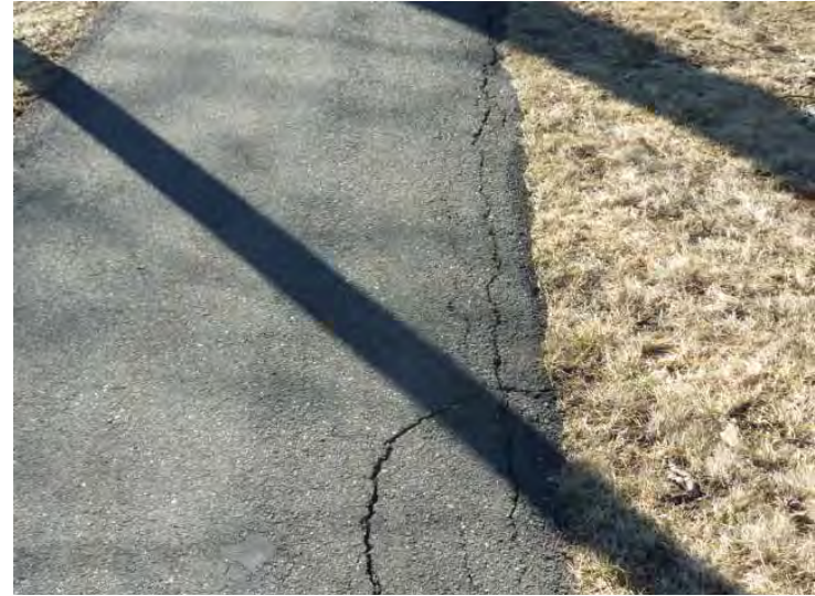
Typical asphalt walk paving has edge failures due to inadequate sub-base.
