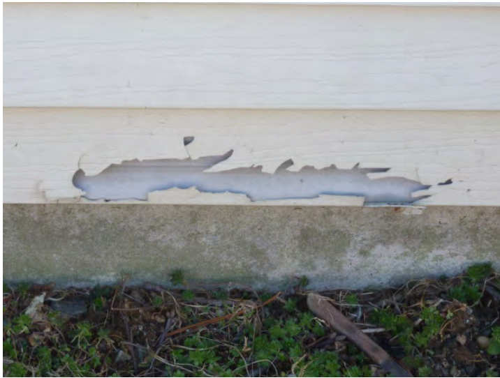
Typical vinyl siding damage.
