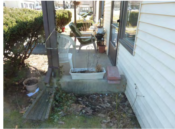
Concrete stoop at designated accessible unit is not accessible.
