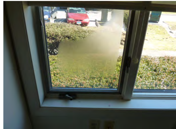
Typical condensation in-side the insulating glass due to seal failure.
